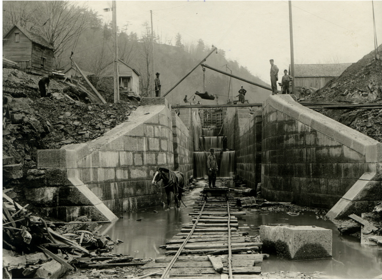
This is the set of the 5 locks on the Black River Canal being built. This photo is in the Erwin Library in Boonville.
